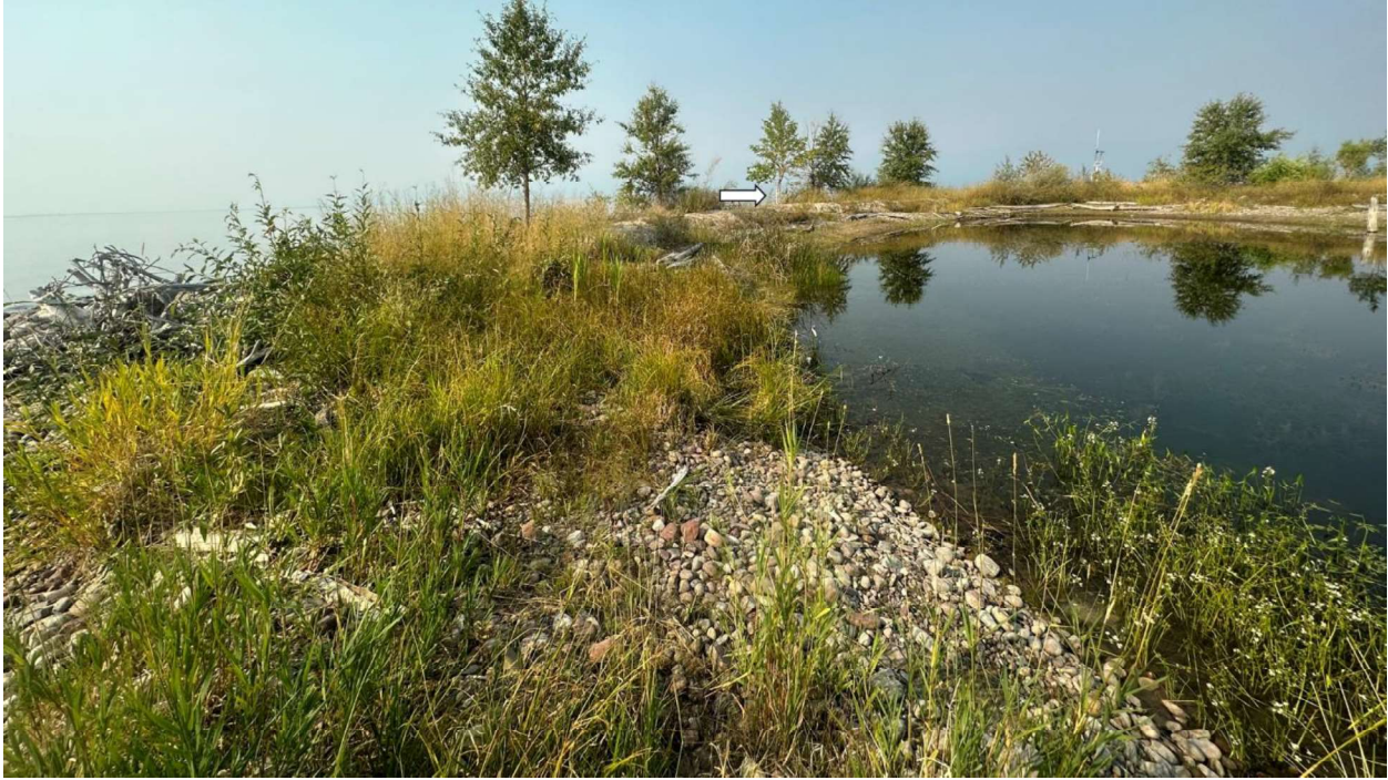
Figure 65. This photograph shows the condition of the 2023 backshore of the gravel dike and spit embayment. The white arrow shows figure 64 view where a break could happen as described in the figure 64 legend.
