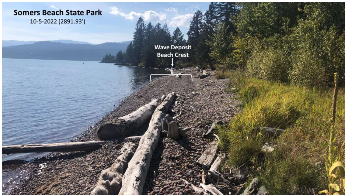
Figure 27. This photograph is of the swimming beach at Somers Beach State Park that corresponds to the survey data shown in figure 26. That material reworked by waves and deposited on top of the constructed beach material is identified by the white bracket which is the beach crest shown in figure 26. This beach crest is the product of the 2022 season of wave power shown in figures 22 & 25.
