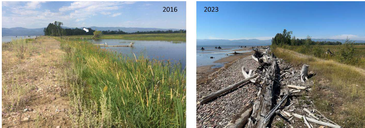
Figure 44. These two photographs together with figure 34 show the change between 2008, the first full pool season after the gravel dikes were built, and 2023. The white arrow shows the position of the willow that appears in several figures as a reference point. The growth of willows and cottonwood trees on the inside of the gravel dike has started the reforestation of the gravel dike. This dike was left to revegetate naturally while the offshore dikes near the river mouth were replanted over most of the dike along the river arm and the spit. This dike would have a more diverse and mature forest had it been replanted with riparian trees and shrubs. Wind blown sand that deposits on top of the gravel helps the natural revegetation process. Foot traffic keeps a path open (Figs, 43 and 44)
