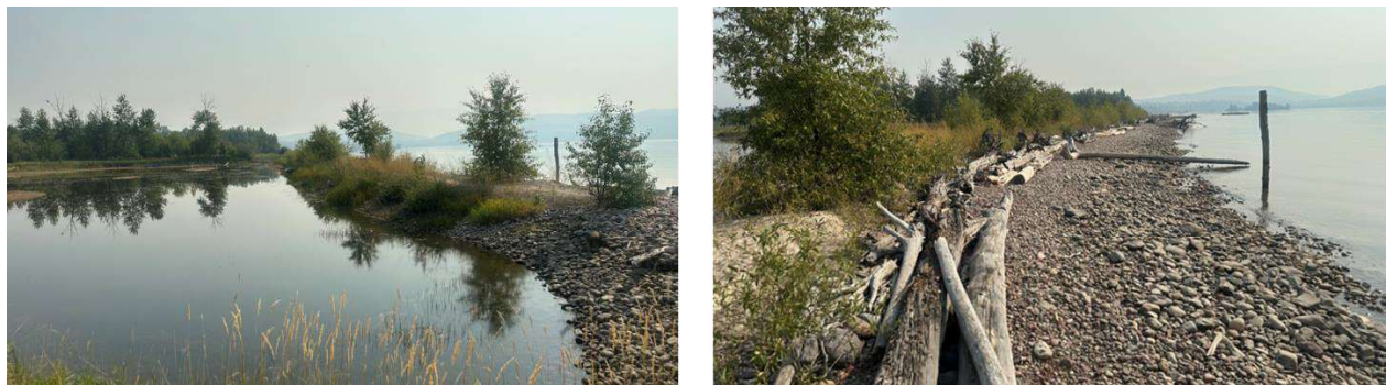
Figure 59. These two photographs show the 2023 shoreline condition of the offshore dike looking east from the spit. The southern wave side maintains a dynamic beach whose job is to extract and absorb all the wave energy (right photo piling G) while the northern pond side is calm enough to allow riparian trees and shrubs revegetate the dike (left photo). Piling G can be seen in both photos. The pilings correspond to transect lines where survey data was extracted from the DEM, and DSM's.
