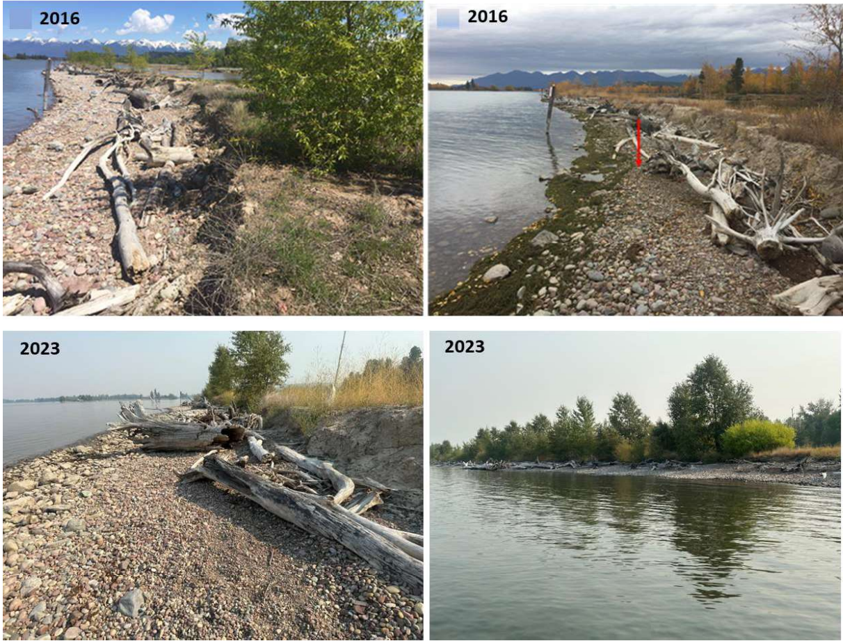
Figure 55. These four ground-based photos compare the change in shoreline condition for the offshore gravel dike and lakeward beaches between 2016 and 2023. The red arrow points to the deposition of aquatic plants by wave action. Although the vertical bank leads one to assume that this area is eroding the actual measured change in shoreline position does not support that assumption. This shoreline is in a state of dynamic equilibrium where waves move and shift the supply of logs and the available gravel creating a shifting habitat mosaic. Leave it alone and if a surface breach occurs here that would be a good thing because it would allow better exchange of water between the lake and the ponds behind the gravel dikes. Piling A can be seen in the top photos.
